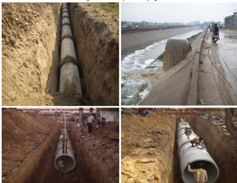
Figure 16 New Pipelines Laying
